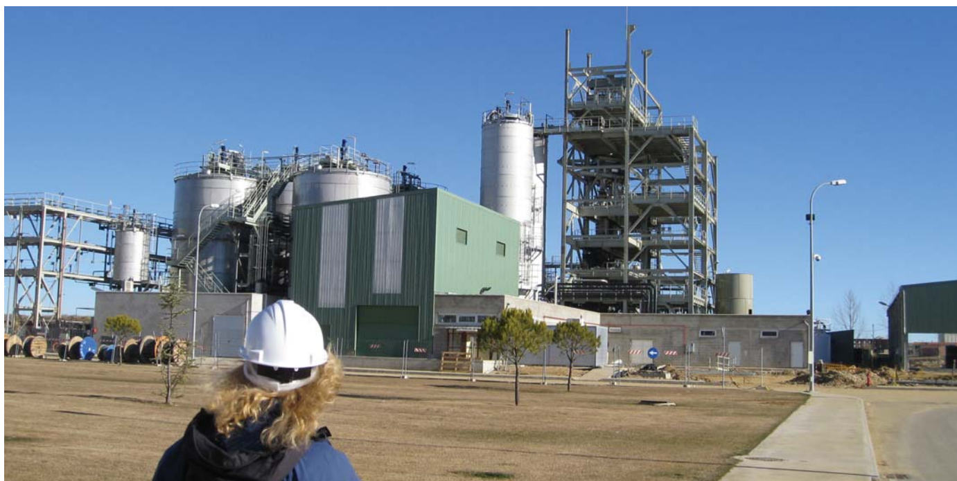
The Abengoa Bioenergy's straw to ethanol demonstration facility in Salamanca, Spain. Courtesy R. Wooley, Abengoa, USA.
