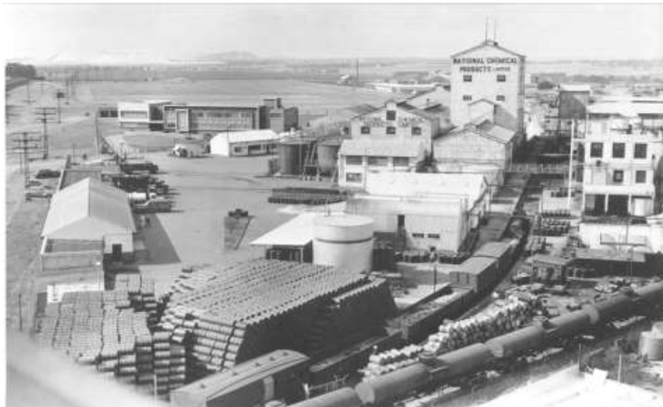
Picture 1: National Chemical Products ABE Facility in Germiston, South Africa
