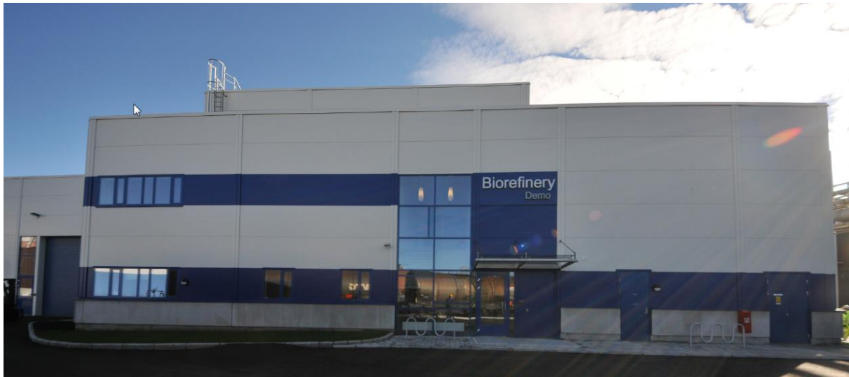
The Borregaard AS Biorefinery demonstration plant in Sarpsborg
