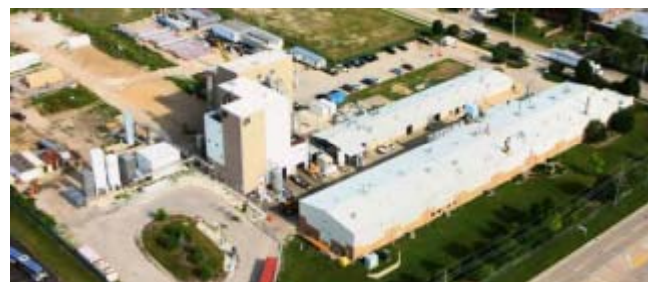
Energy & Environmental Technology Center
