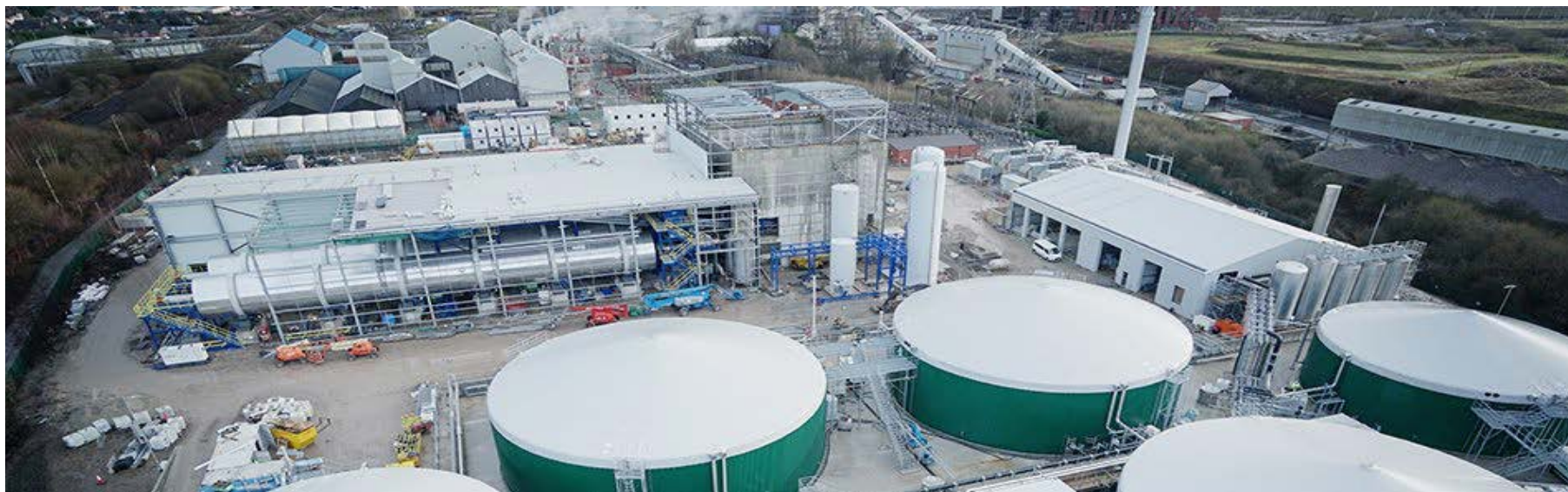
Renescience waste conversion plant Nortwich, England
