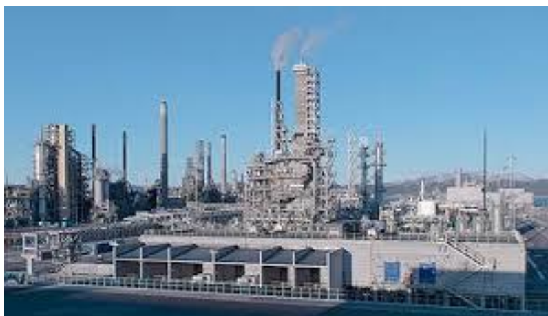
Figure 8. Equinor refinery at Mongstad, Norway. (Photo: Equinor)
